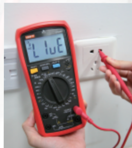
Live and nature wires identification
