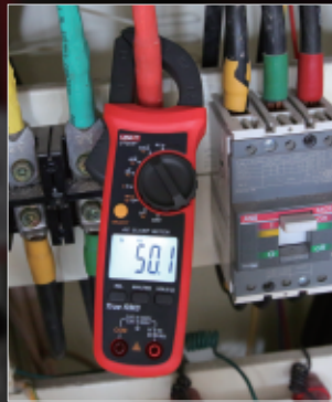
High voltage (600V) frequency measurement
